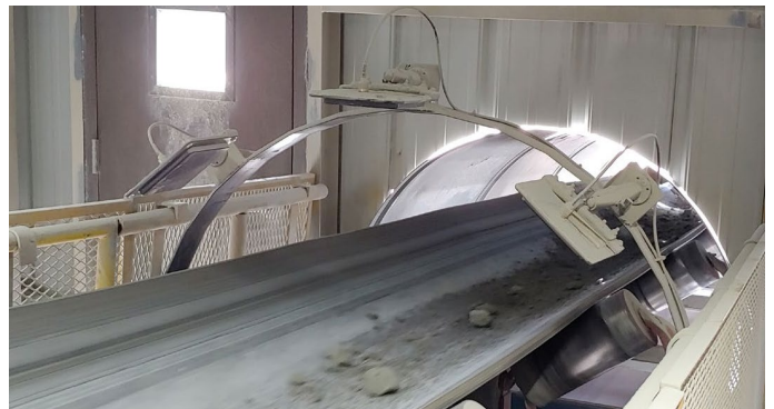
Silo ore belt TopVu installation (skipped ore muck from the shaft).
